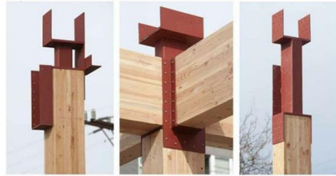
2012-3-8 0210_442_460 Glulam column caps at the Bullitt Center photos: John Stamets
