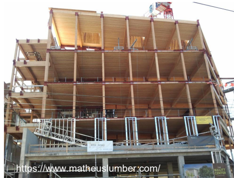
2012-3-8 0210_442_460 Glulam column caps at the Bullitt Center photos: John Stamets
